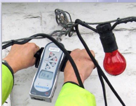
Pull test on anchorage points
