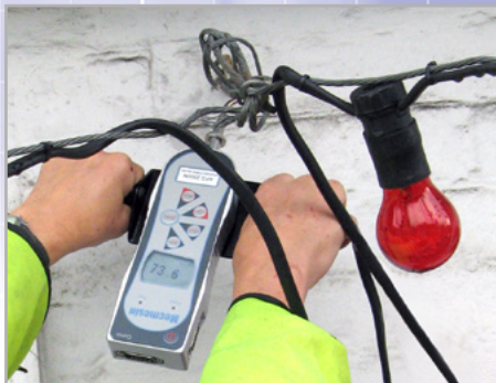
Pull test on anchorage points
